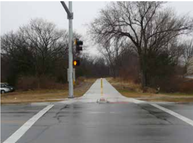
Hybrid Beacon. The hybrid beacon (or HAWK signal) functions somewhat like school bus warning signals. It is dark when not in use. When actuated by a pedestrian, a flashing and then solid yellow light warns motorists to slow; a solid red light paired with a walk signal stops traffic and gives the right-of-way to the pedestrian. Users report a high degree of motorist compliance and a positive effect on pedestrian safety.
