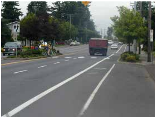
Midblock Refuge Medians. A crossing median provides refuge to trail users at mid-block crossings, reducing the distance that pedestrians and cyclists are exposed to traffic.
