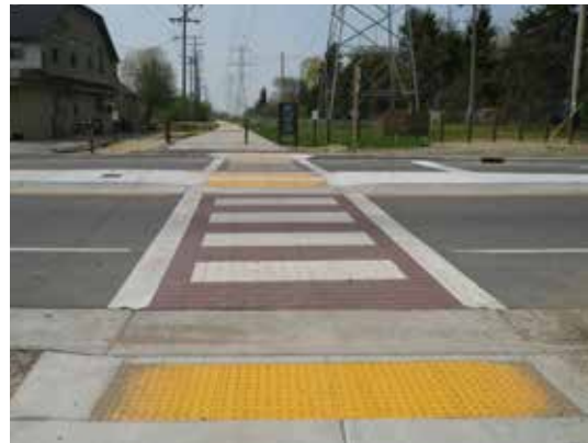
Contemporary trail crossing. This crossing of a major arterial includes a refuge median, defined crosswalk, effective warning signage, and the consultant's bike.
