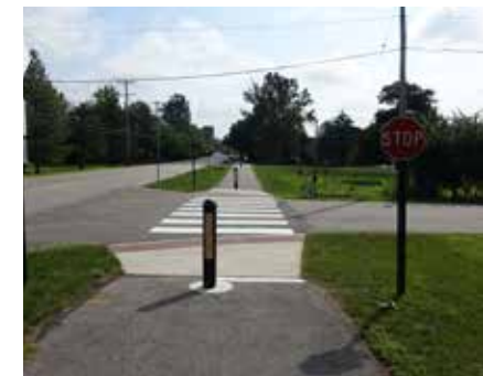
Good sidepath intersection design: Ramp is directly in line with travel path, crosswalk is unobstructed and clearly marked.
