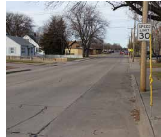
Washington Avenue, a key north-south corridor in Great Bend. The street’s typical 48-foot width is adequate to maintain parking and add bike lanes.
