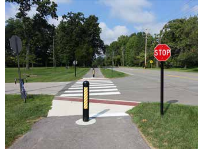
Sidepath with well-marked crossing, Clayton Road in Saint Louis County, MO
