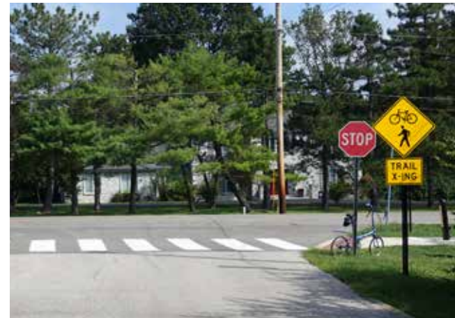
Sidepath Advisory Signs. Top: Variation of the MUTCD's Railroad Advance Warning Sign, modified as a sidepath advisory. This sign should be used on both sides of a road with sidepaths. This installation is on Speer Boulevard in Denver, advising of the parallel Cherry Creek Trail. Florida DOT advises a similar sign. Above: Trail crossing advisory sign on an intersecting side street, installed on Clayton Road in suburban Saint Louis.
