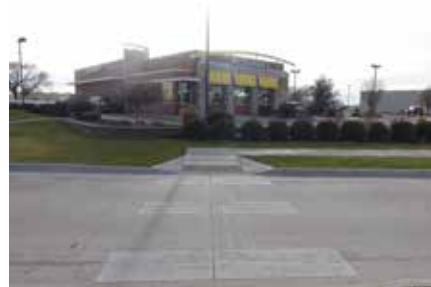
Ladder Crossing at 10-Harrison intersection
