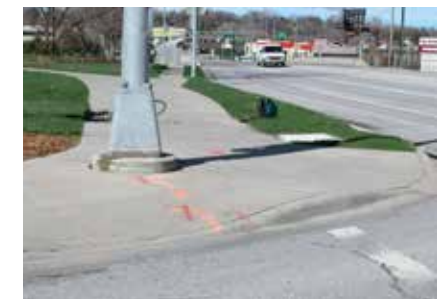
Poor Sidepath Intersection Design. Top: Ramps are narrow and located off line from a bicyclists normal path, creating a potential hazard. Above: The base of a signal mast arm obstructs the logical path through the ramp.
